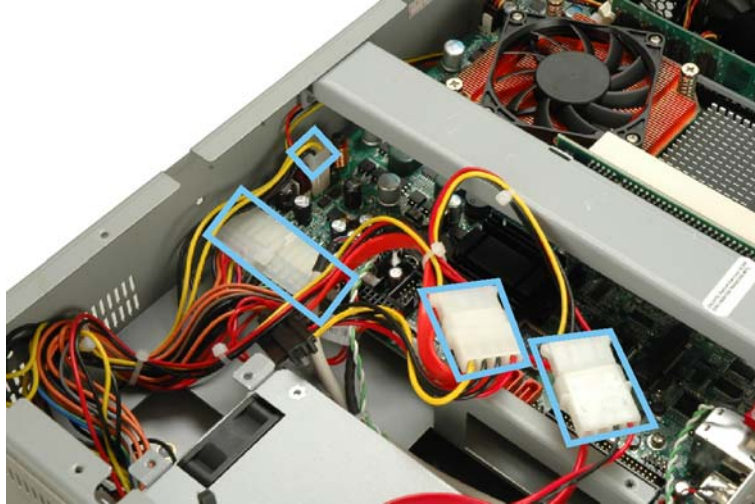
Figure 7-6: PSU Power Cables
